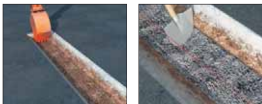
Setting the channel, haunching and filling in
